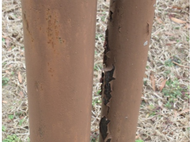
Finish deterioration
