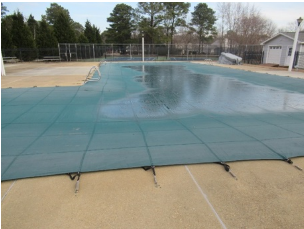
Main pool overview
