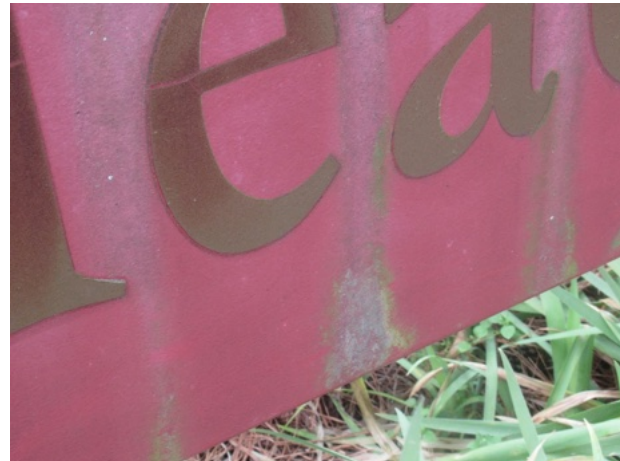
Metal finish deterioration
