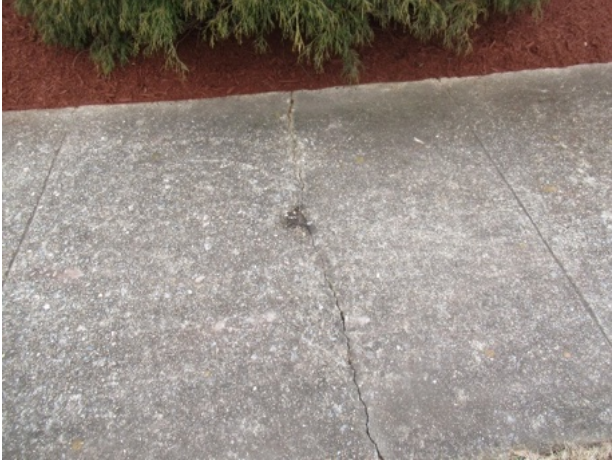
Sidewalk crack
