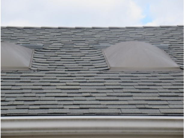
Pool house roof overview (note skylights)
