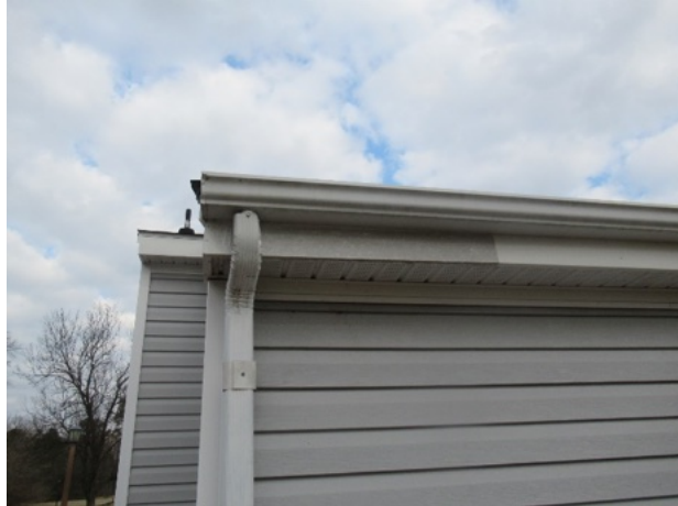
Typical gutters and downspouts
