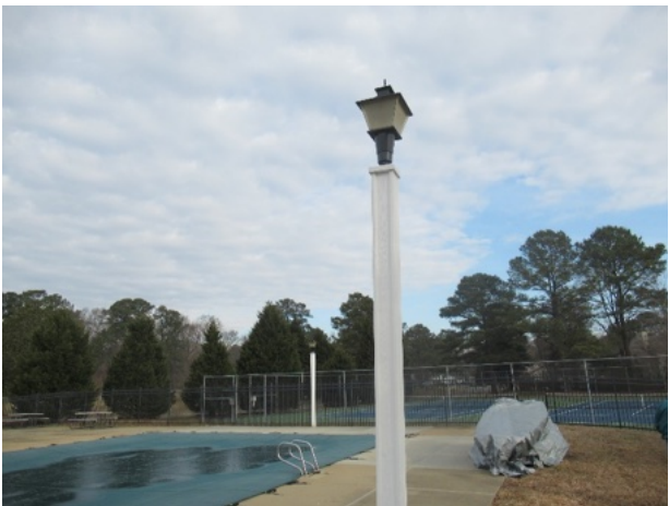
Typical wood light fixture
