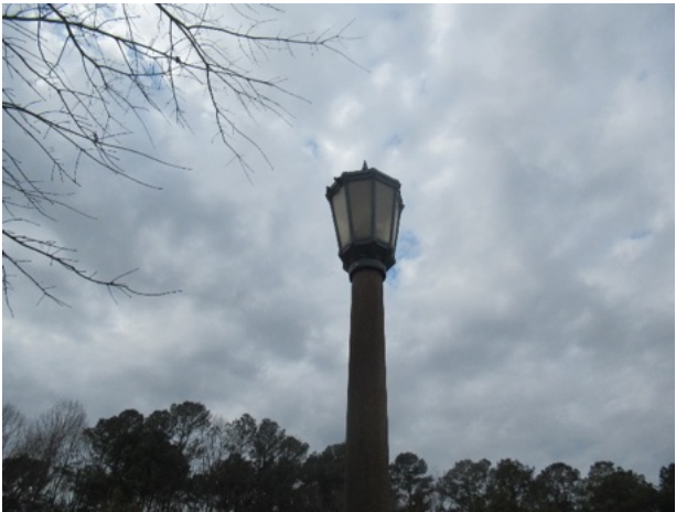
Typical concrete light fixture
