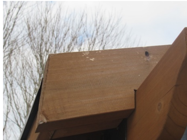
Finish deterioration
