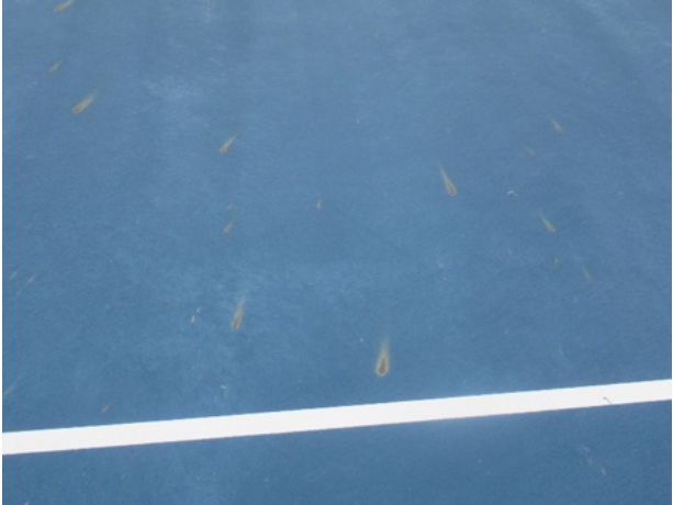
Paint deterioration
